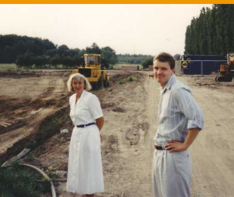
New factory building
